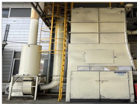
[Filter Dust Collectors in the R&D Center]
